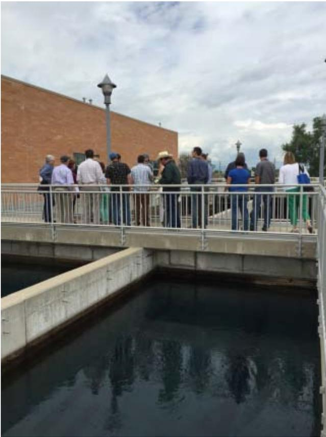
conveyed to large tanks where chemicals are added that make suspended particles clump together. The clumps settle to the bottom and the clear upper layer is drained
